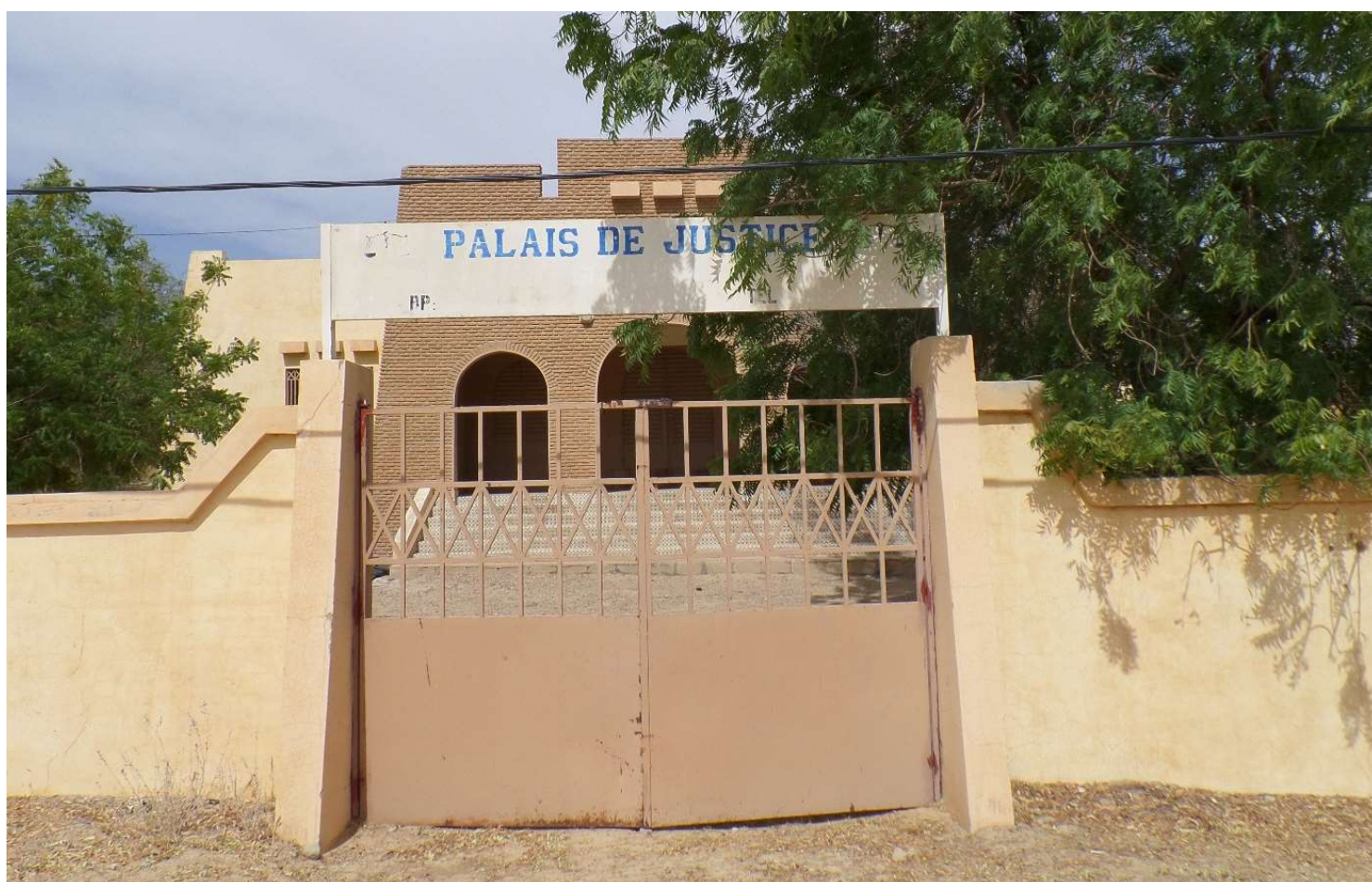
Courthouse in Mali Photo: JCS
